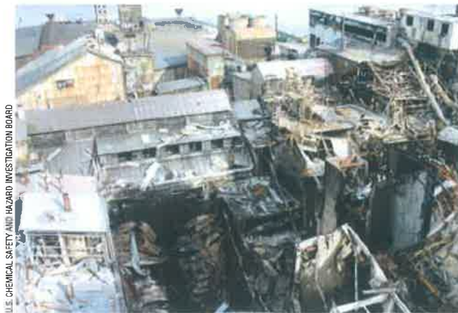
Aftermath of the February 2008 dust explosion and fire at Imperial Sugar refinery in Port Wentworth, Ga.
